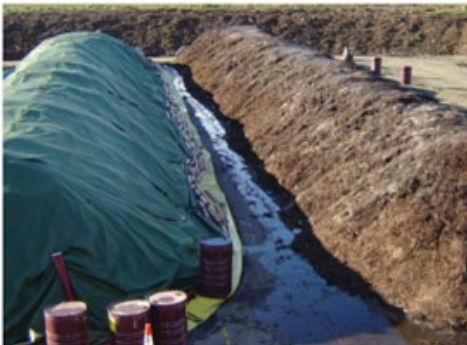
Windrow mounted spray systems for Compost Turning
