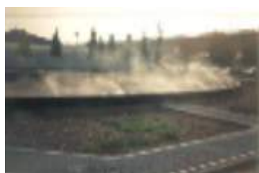
Figure 4.2: Paper industry wastewater plant surrounded by nozzle system misting Ecosorb®
